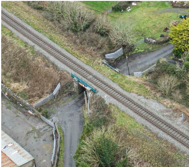
Stone bridge at L71051
