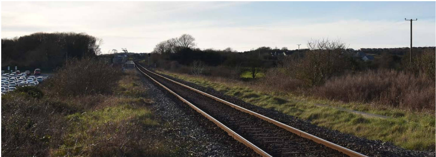
Single track rail line looking west towards Galway
